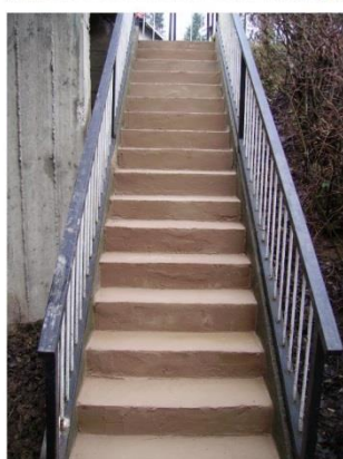
Stairs repair at minus 9 C
