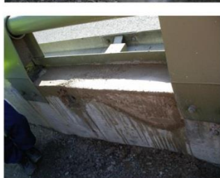
Repairs of concrete damaged by salt
